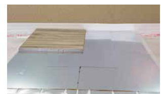
8. Laying of surface finish (floating on special mat recommended)
