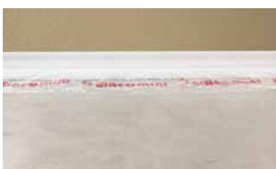
1. Laying of wall edging strip
