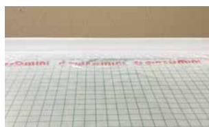
2. Laying of steam barrier polyethylene sheet
