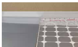
6. Positioning of first galvanized steel sheet layer
