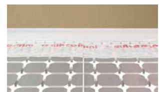
4. Laying of R883-1 insulation panel with coupled aluminum heat transfer profile
